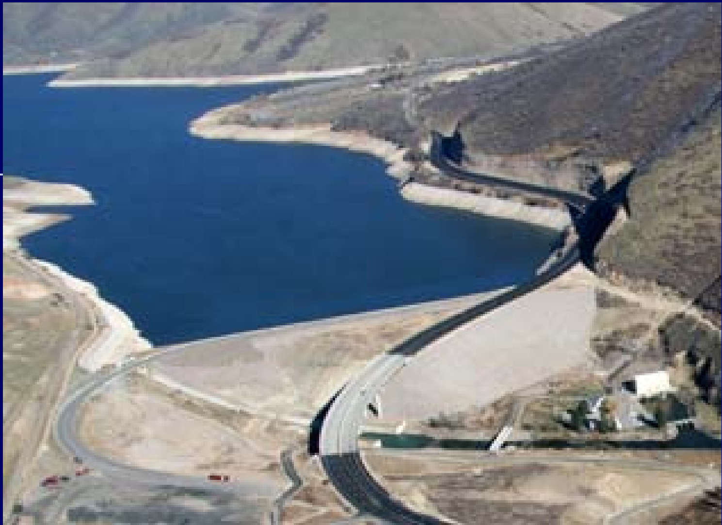
Remediated Deer Creek Dam with realigned state highway across downstream slope (U.S. Bureau of Reclamation photo)
