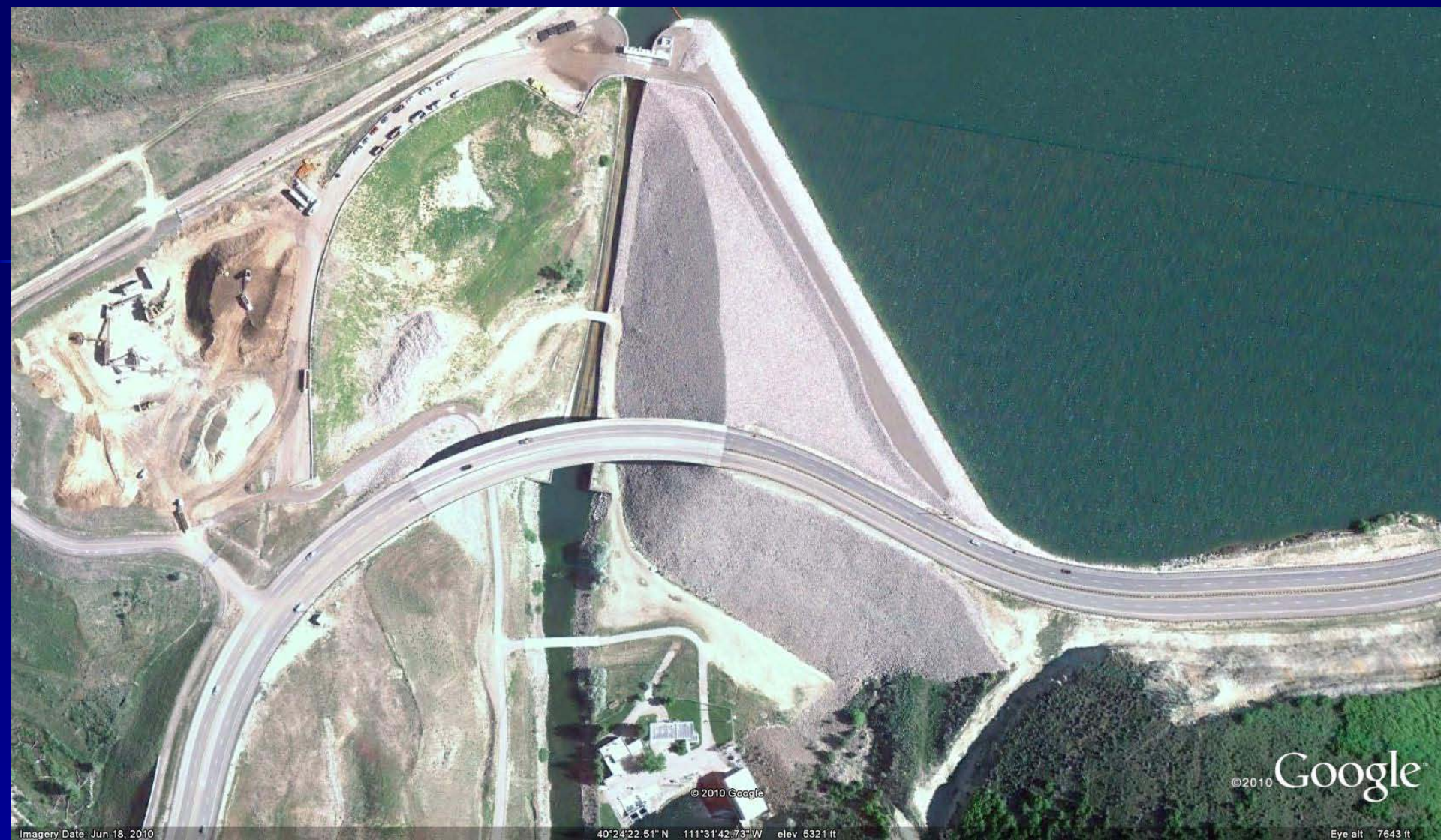
DEER CREEK DAM, Utah: Remediated using Downstream Shear Key and Berm; State Highway relocated over Downstream Embankment Slope
