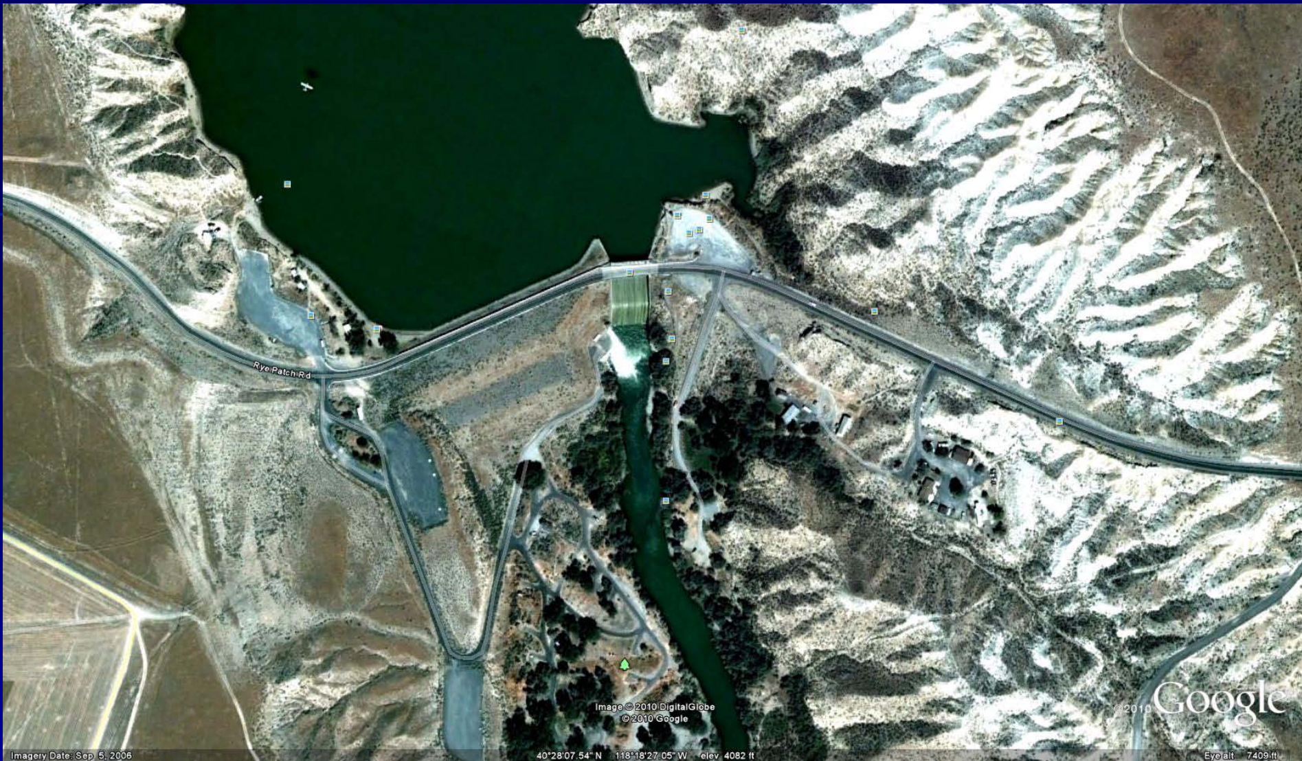
Rye Patch Dam, NV: Remediated in late 1980's using a Soil-Cement Key-block and Downstream Overlay Buttress Fill
