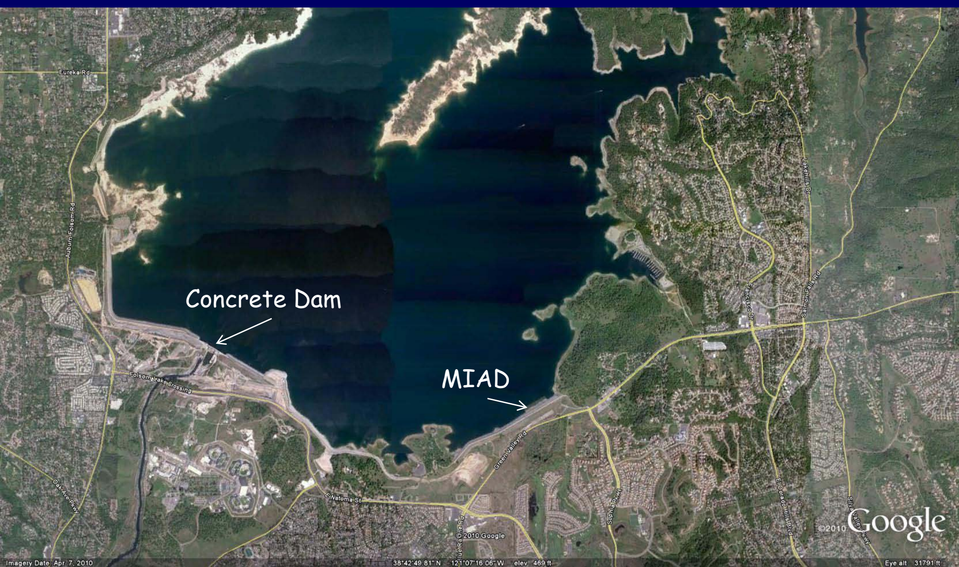
FOLSOM PROJECT: Concrete Main Dam with Embankment Wing Dams, Mormon Island Auxiliary Dam and 8 Dikes
