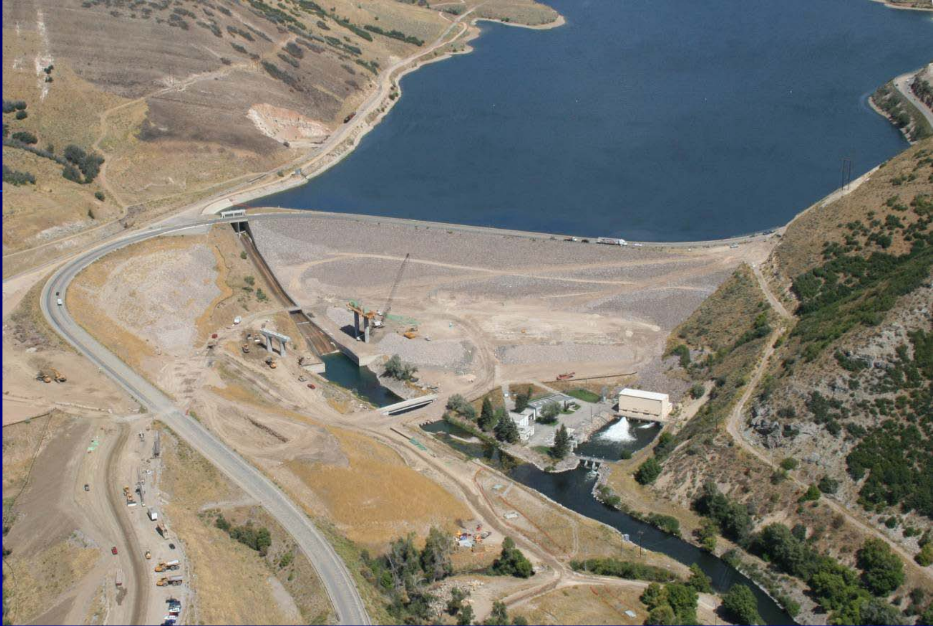
Pier construction for relocated Hwy 189 on DS face of 90 remediated Deer Creek Dam
